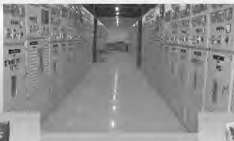
3.6 kV TO 12 kV INDOOR CIRCUIT BREAKER PANEL Ratings : 12 kV up to 3150A, 40 kA
