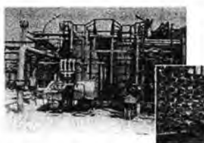
Effluent recycle plant at a fertiliser factory
