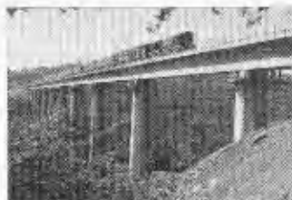
One of Asia's highest viaducts built by L&T
