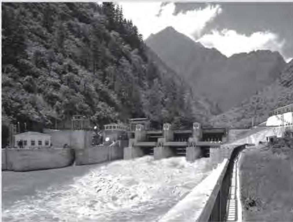
400 MW VISHNU PRAYAG H.E. PROJECT
